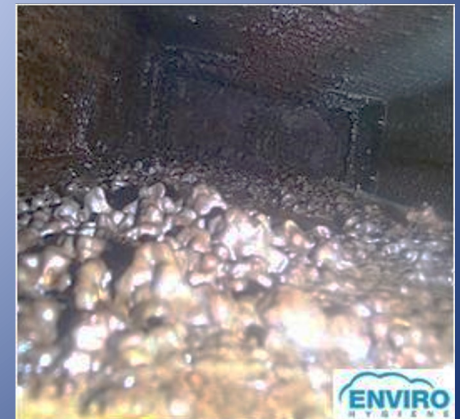
Grease in Duct Close-up
