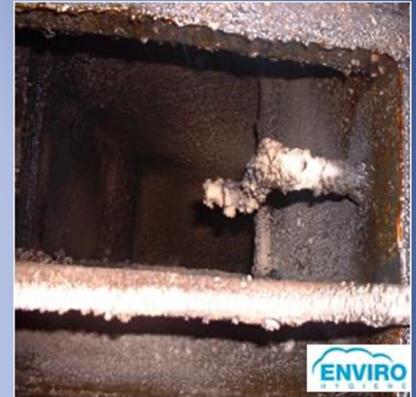
Duct component covered in Grease
