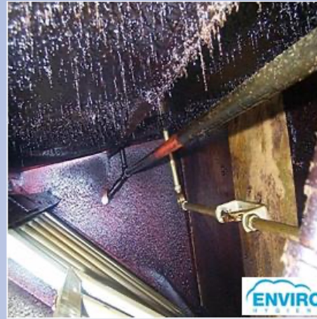
Behind the Canopy Filters
